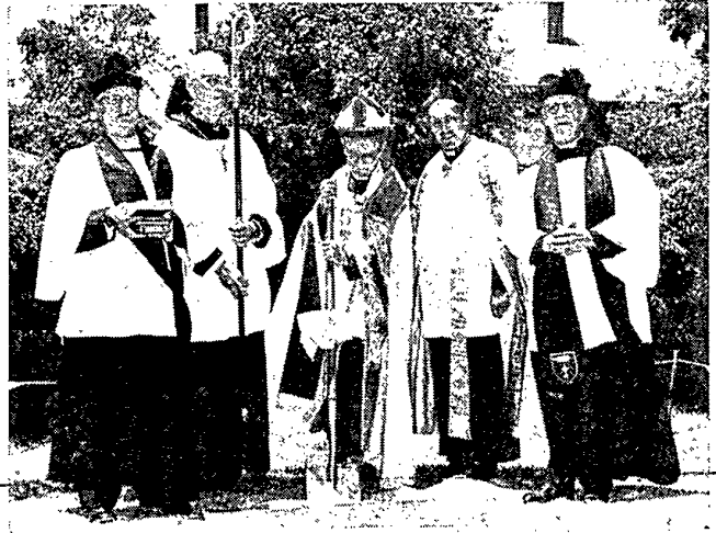
New church building started at Ormond Beach.
